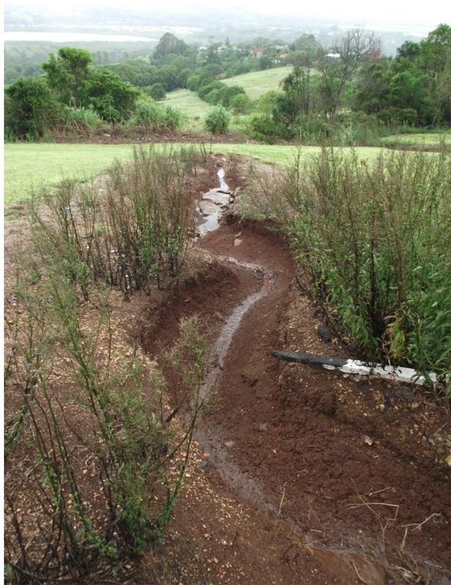
**Figure 6 – Existing Scoured Drainage Line below Pipe under Terranora Road**
